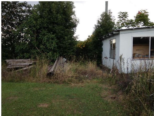
Looking south around the eastern end of the existing shed in the southeast of the site
